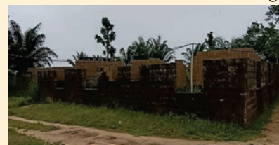
Alumni Building Under Construction
