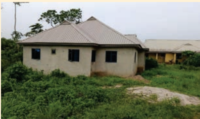
3-Bedroom Flat Under Construction by Lagos Conferences
