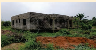
Rector's Lodge Under Construction by Yaba Baptist, Lagos.
